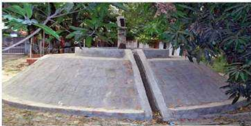
Figure 36: Pompe à main anti-inondation
